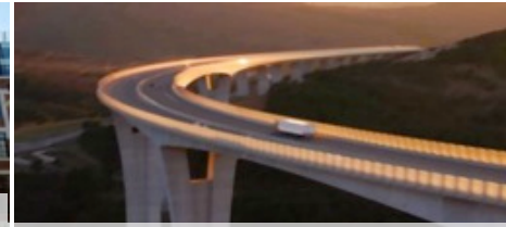
KRINKAL BRIDGE - SLOVENIA
